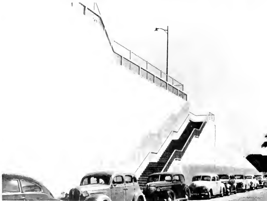
Looking southeasterly, showing portion of retaining wall and stairway construction on east side of Oak Street to provide passenger interchange between bus stop above and city street below
